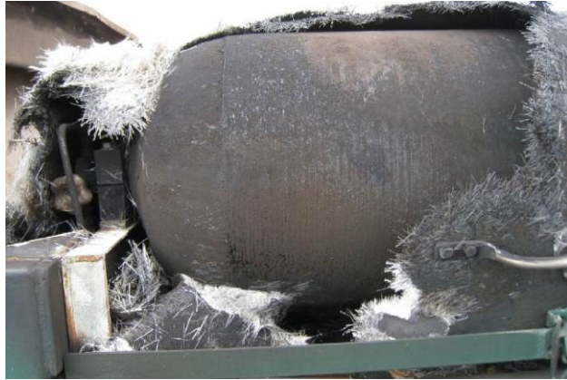
Figure 31 Fire damage. In this photo, the outer composite cover has burned away. The cylinder, although intact, must be immediately inspected by a CGA C6.4 certified or other qualified CNG inspector.
